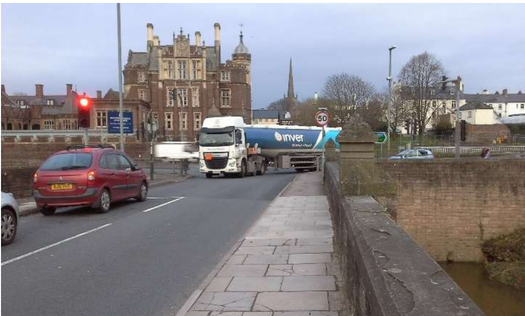
Plate 8 - View West along the Wye Bridge showing the impact of Heavy Goods Vehicles turning onto the bridge, which inevitably causes the Heavy Goods Vehicle to swing towards the pedestrians and cyclists whilst re-aligning to the carriageway. Both carriageways are significantly below current standards. The impact on the paving system of vehicles mounting the curbs can be seen in the cracked paving.
