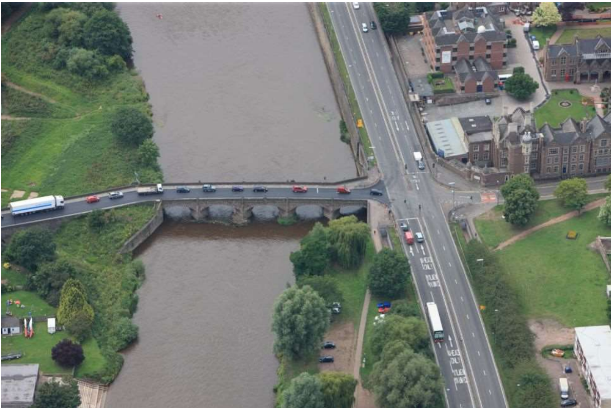
Plate 6 – View of the Grade II listed five span arch masonry Wye bridge
